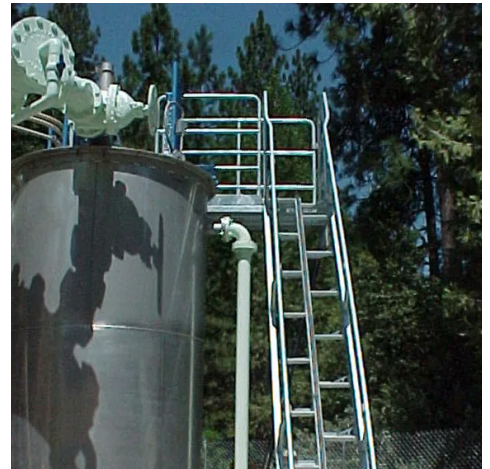
TANK & SILO ACCESS
