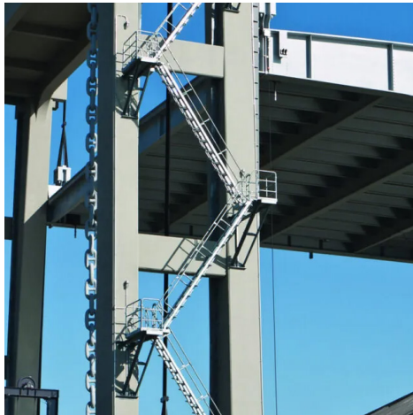
STAIR TOWERS — HIGH-RISE ACCESS
